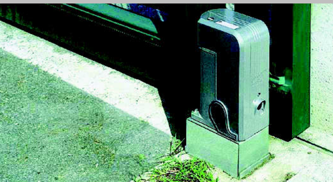
Installation of the operator
